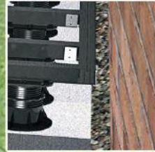
Frame starts 15mm away from wall
